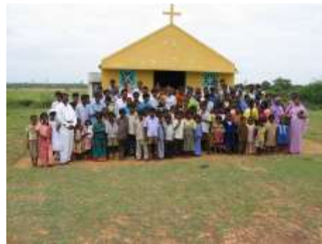
This church in India (steel girders and concrete block) costs $7000 to build.
